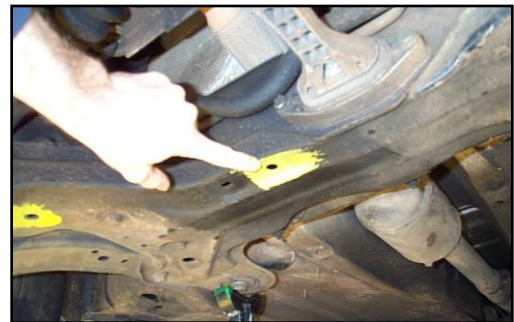
Figure 31 - Center 13mm Hole Pre-Drilled In the Subframe
